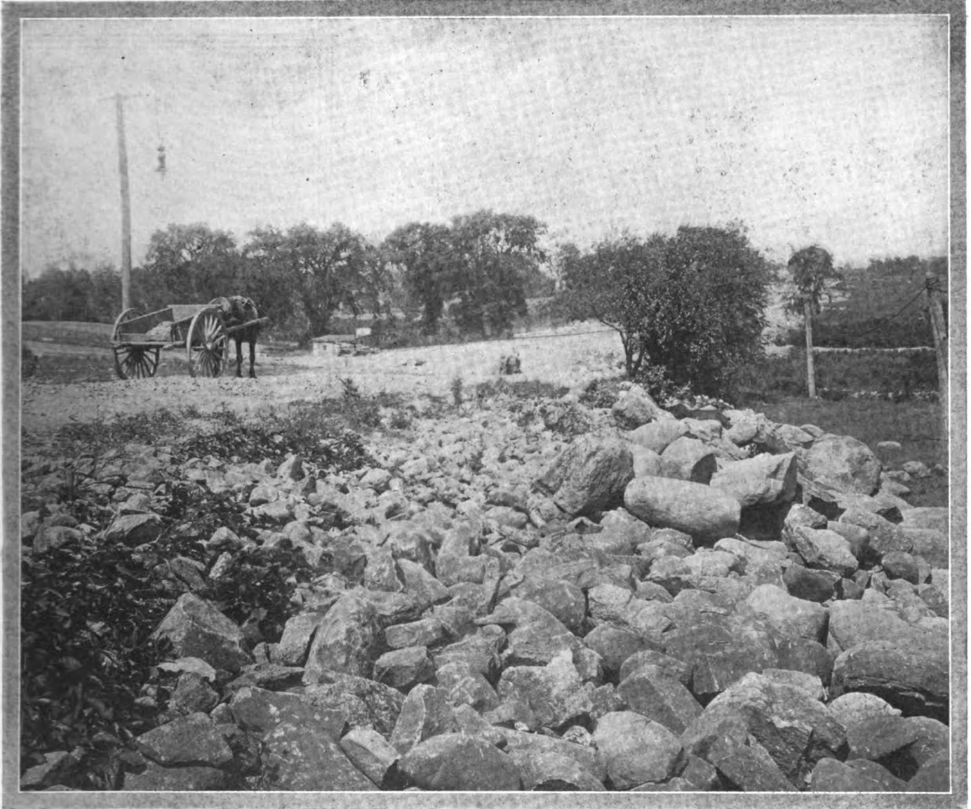
L—In widening the Boston Post Road boulders are being used to form a roadbed and the illustration depicts the heterogeneous class and size of material being employed. It is proposed to widen the road to the posts seen on the right-hand side of the picture
